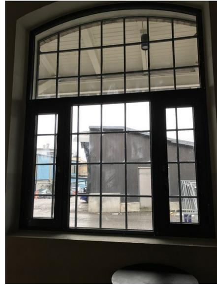
*The external window is original and the inner window with an u-value of 0,6 was installed*
