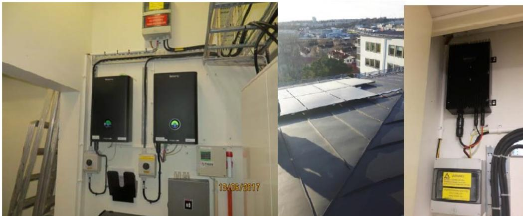
*EnergyHub inverters (left), PV cells (centre), and control system (right)*
